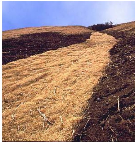
Figures 6.20-7 and 6.20-8. Examples of Compost Blanket (Filtrexx) and Permanent Erosion Control Jute Matting (North American Green website)
