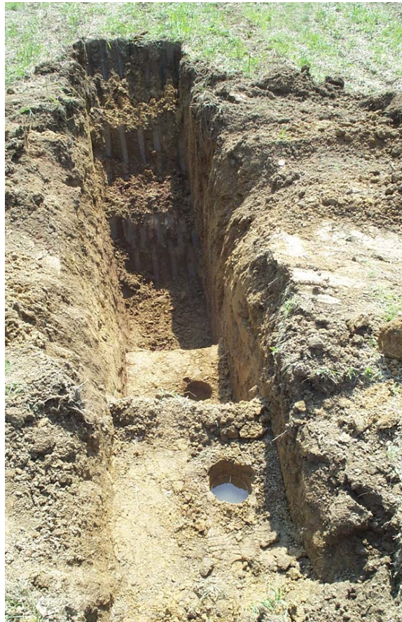
Figure 4 Deep hole with multiple benches
