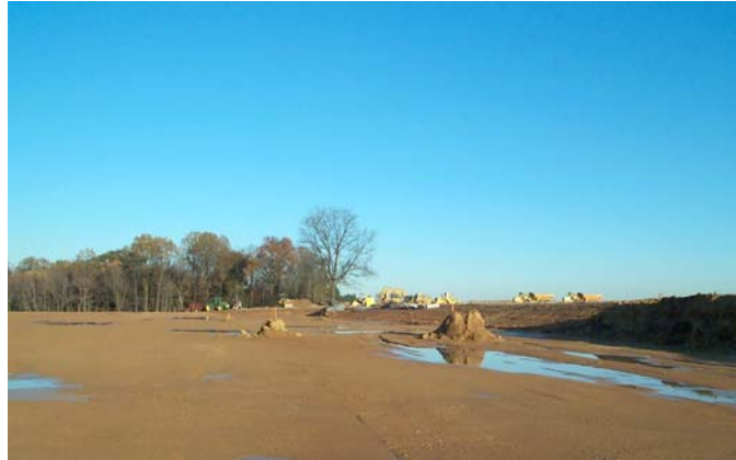
Figure 6.19-1. Soil compaction and cutting during construction.
