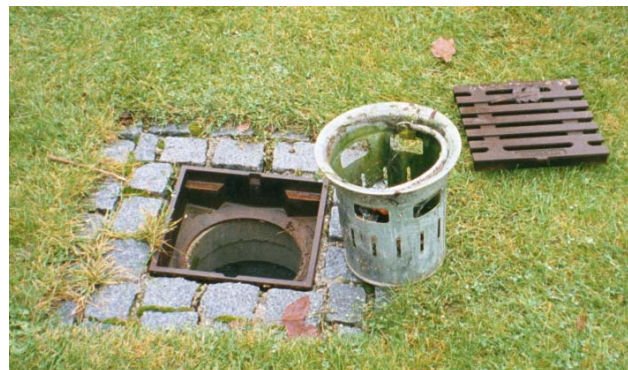
Figure 6.16-4. Example of a german basket-type water quality inlet, (CA, 2001).
