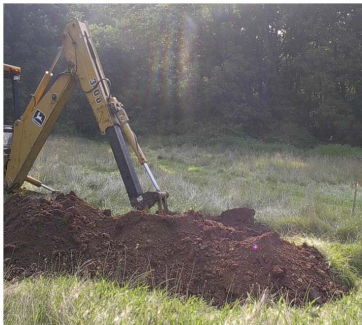
Figure 3 Excavation of deep hole by backhoe
