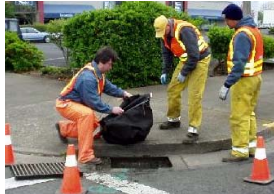
Figure 6.16-3. Filter Bag Installation (Full Circle Ag, Inc., http://www.fullcircleag.com/pages/954364/ )
