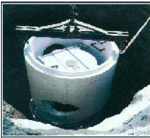
Figures 6.16-6. Vortex separator ( http://www.hydrointernational.biz/nam/ind_storm.html )
